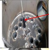
Boiler cleaning brush inserted into heat exchanger tubes
